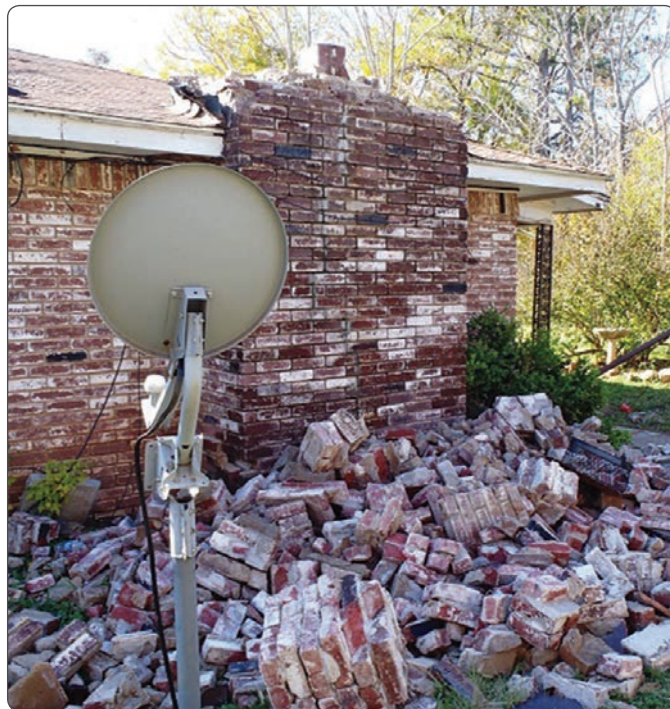
Residential damage from the magnitude 5.7 earthquake in 2011 that struck Prague, Oklahoma. PHOTO BY U.S. GEOLOGICAL SURVEY
